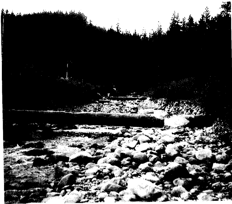
Figure 19: Oulette Creek 1982, Howe Sound, BC. In the first three years following channelization, the single log drop structures added to the uniform channel were undercut. Alternating single boulder drop structures were buried in deep scour holes formed immediately below the structure crests as there was no downstream riffle to convey the flows away from the structure.
