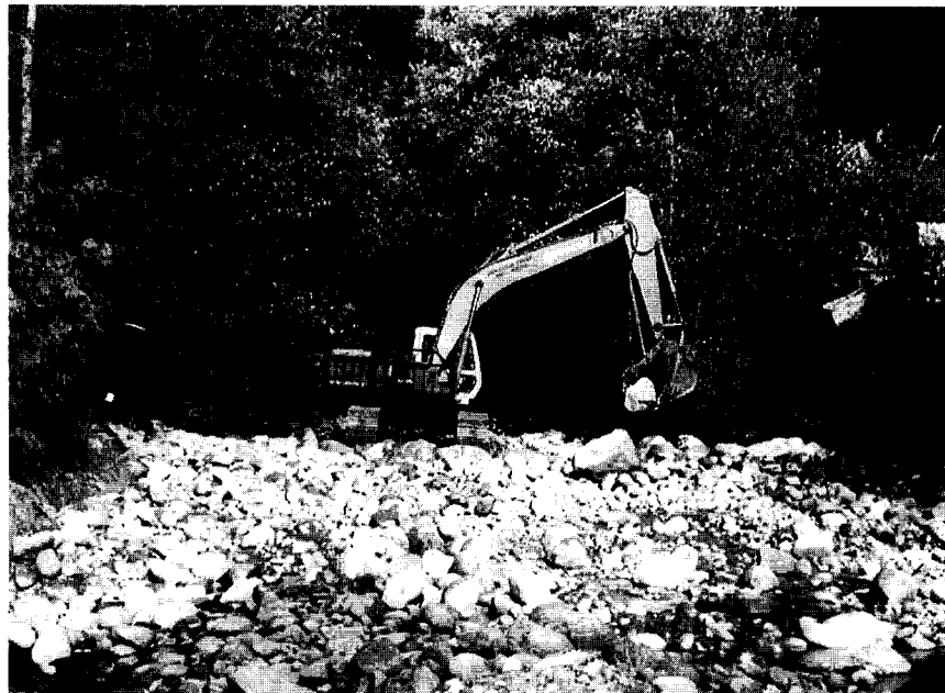
Figure 15: Twin Creek Restoration Project 1993, Howe Sound, BC. Following the steps in the schematic construction drawing (Figure 14), the backhoe operator is sorting and placing the larger boulders along and below the riffle crest. The hydraulic thumb attached to the bucket allows boulders to be moved and placed individually.
