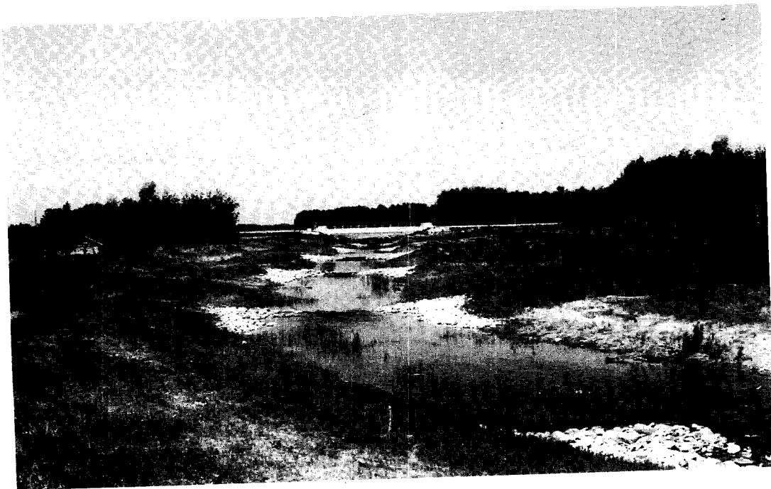
Figure 17: Mink Creek Walleye Spawning Restoration Project 1988, Central Manitoba. The channelized reach 3 years after rock riffles were added. After several bankfull and greater flood events formed downstream pools, the channel has stabilized. The riffles and upstream pools are utilised by spawning walleye.
