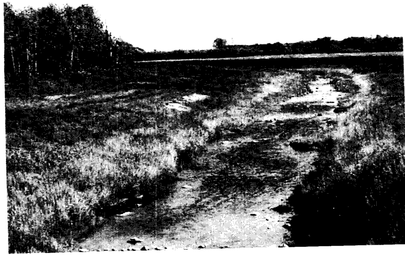
Figure 1: Mink Creek Walleye Spawning Restoration Project 1985, Central Manitoba. The channelized and unstable reach prior to the addition of rock riffles.
