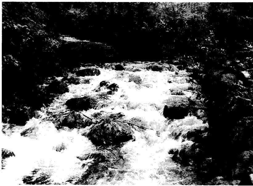
Figure 13: Langdale Creek Restoration Project 1995, Howe Sound, BC. Diverse hydraulic conditions have been created by strategically placing large boulders on the downstream face of this constructed riffle. Note the well rip-rapped banks in the riffle zone adjacent to the re-constructed Sunshine Coast highway.
