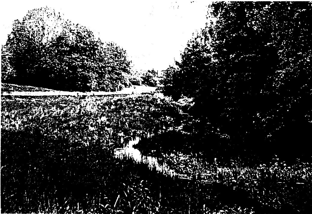
Figure 2. Stretch of Whittle Brook after rehabilitation scheme.
