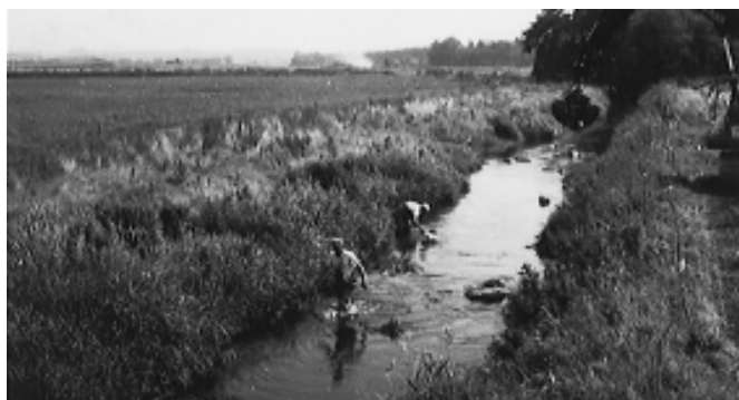
Laying out stones in a two-step profile.
