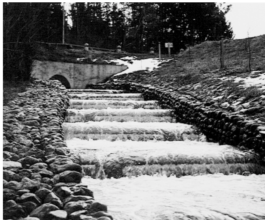
The basin ladder in Græse stream viewed facing upstream towards the road culvert.
