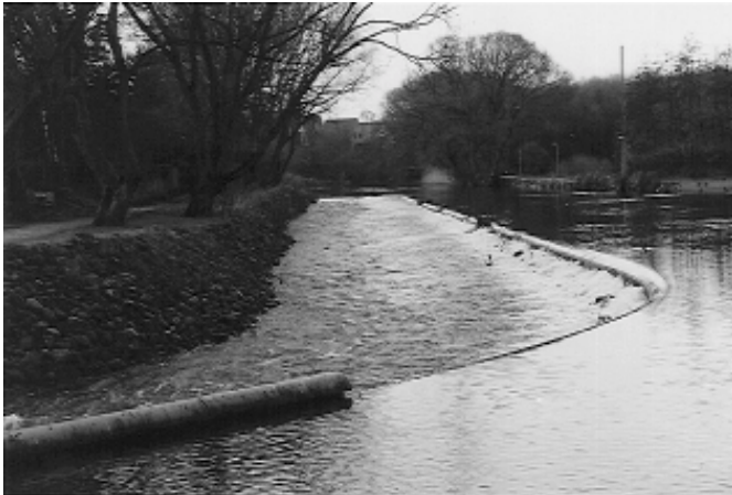
Riffle and spillway viewed facing upstream from the floodgate.
