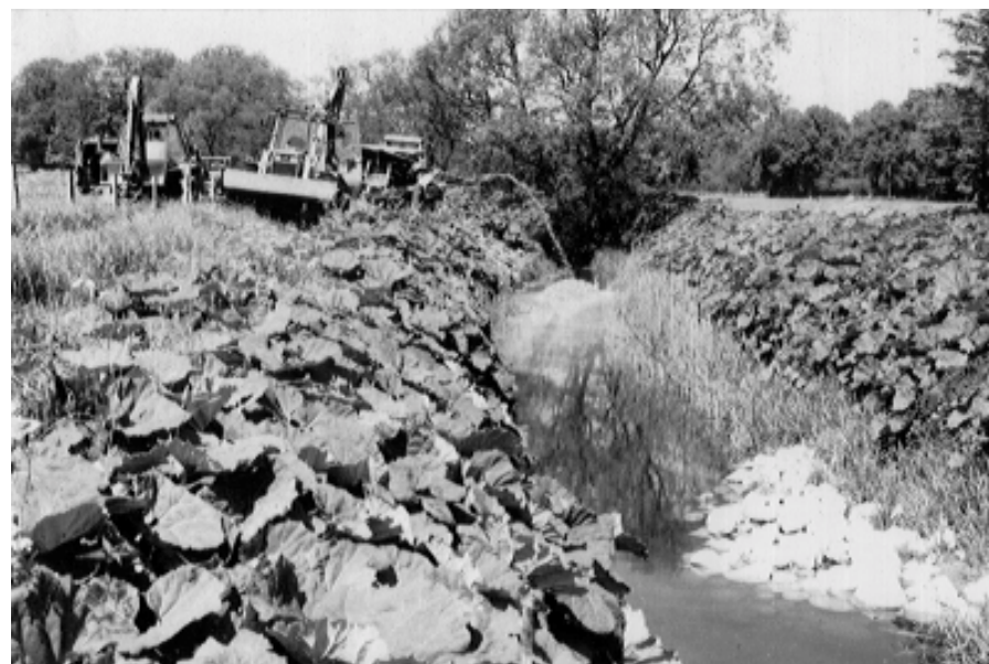
Laying out stones and spawning gravel in Køge stream.
