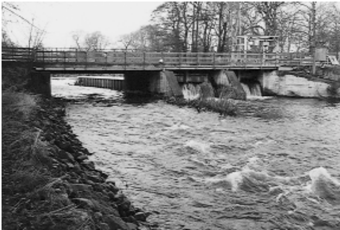
The riffle and floodgate viewed facing upstream from the lowermost resting basin.
