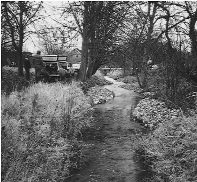
Figure 4.7. Current concentrators – made, for example, by placing mounds of coarse gravel on alternate sides of the watercourse – ensure that the current is strong enough to keep the gravel banks free of sand.
