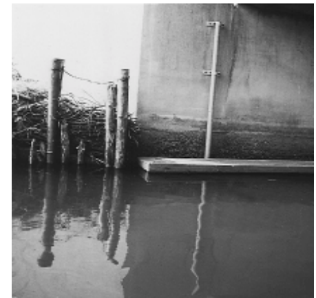
Figure 4.16. Otter pass. This is a type 2 rehabilitation method that helps otters to pass under bridges. Many otters are killed by vehicles in Denmark when trying to cross roads over streams.
