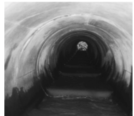
Figure 4.13. Current breakers in underpass culverts. In order to enable fish to pass through a culvert one can raise the stream water level and insert current breakers.
