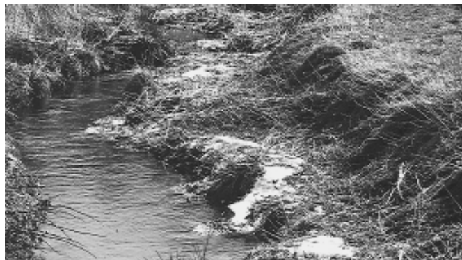
Figure 4.3. A two-step cross-sectional profile ensures an adequate water depth and current in dry periods.
