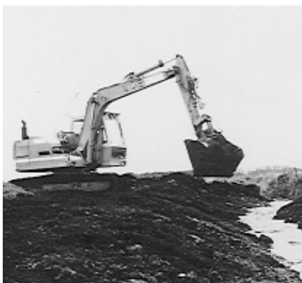
A new watercourse being excavated.
