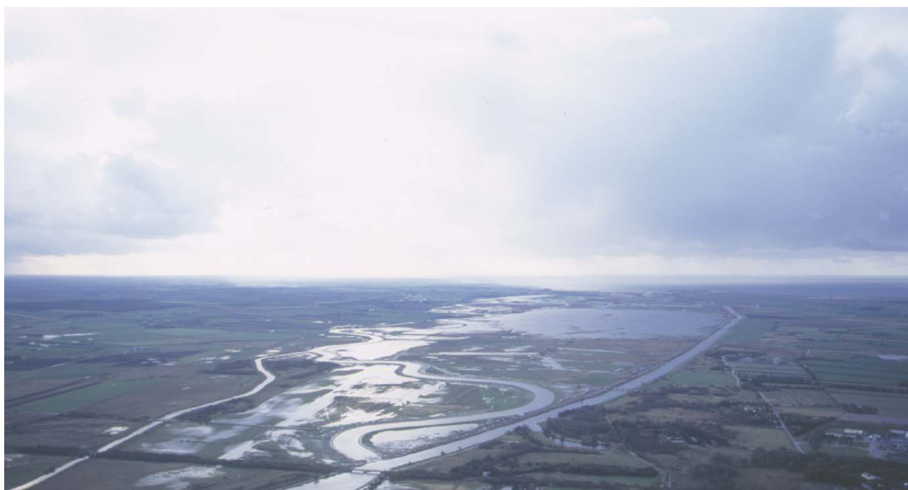
Restoration of river Skjern, 2002.
